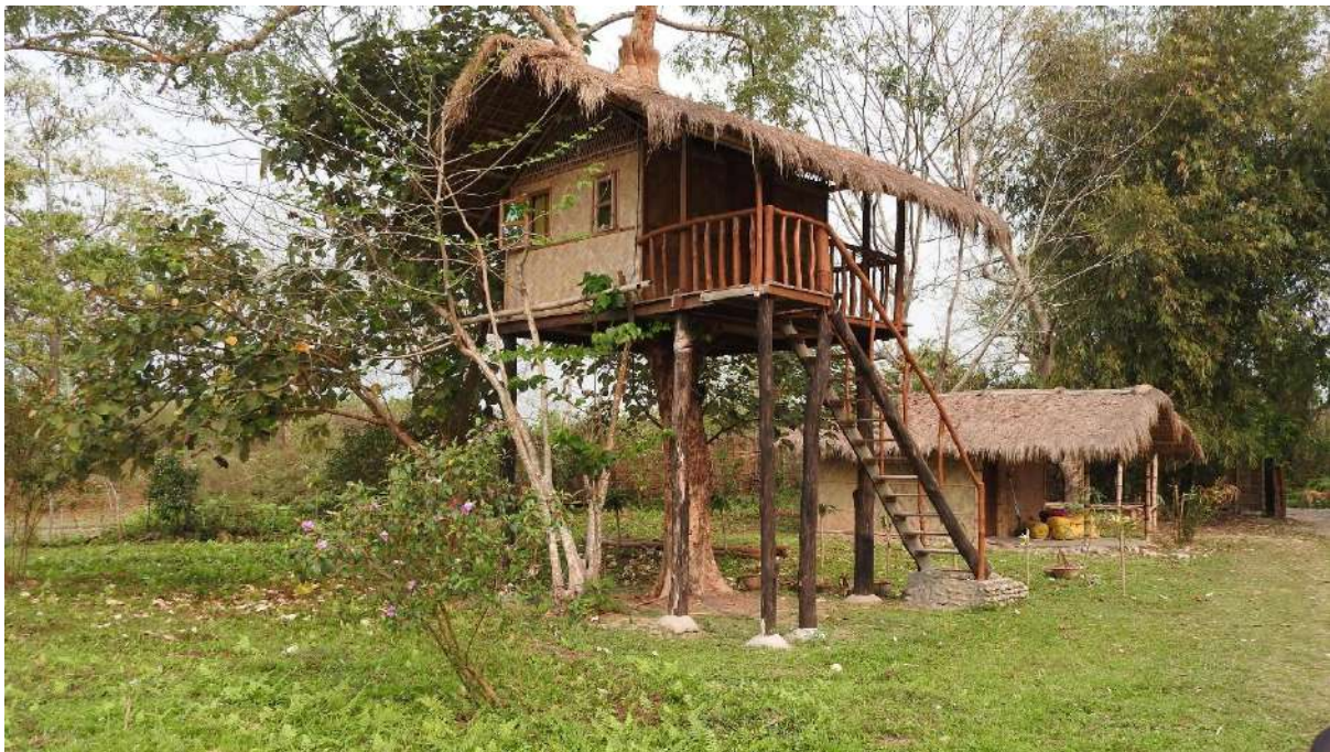
Fig 7. Tourist tree house cottage built by Mr. Pratap Das in Nameri
