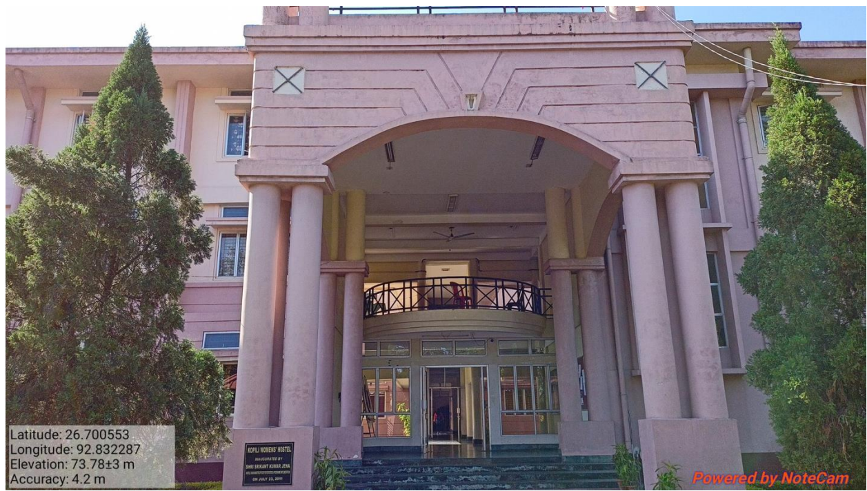
Outdoor view of Kopili Womens' Hostel
