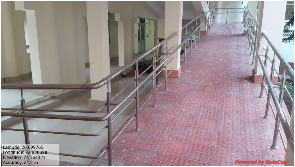
View of a Ramp
