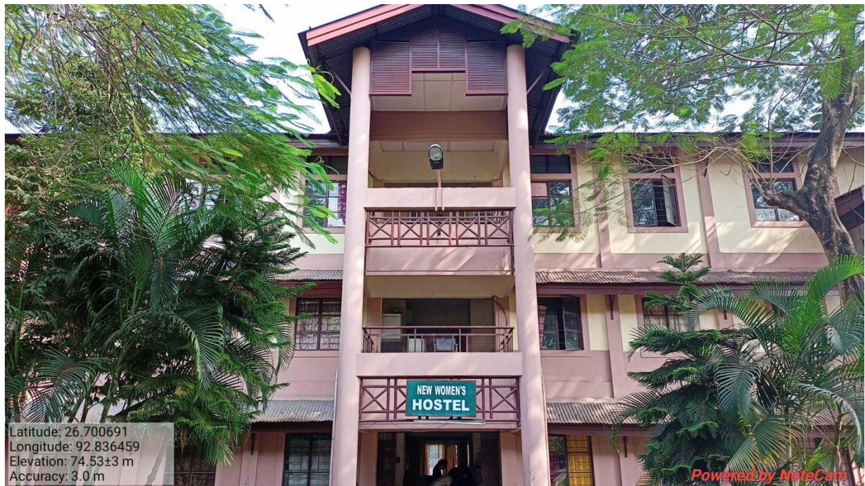
Outdoor view of New Womens' Hostel
