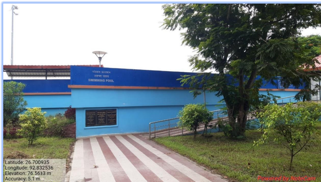
Front view of the Swimming pool
