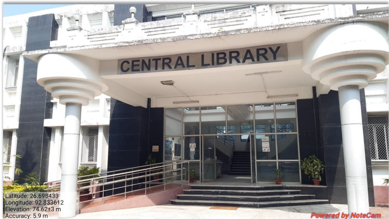
Front view of central library
