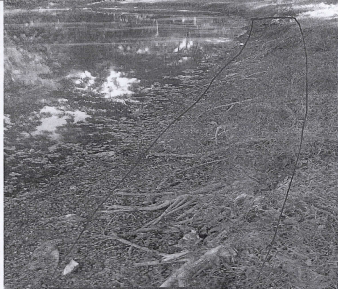
SOIL EROSION IN THE BANK OF THE WATER BDOY LOCATED IN FRONT OF HSS BUILDING
